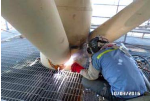
Gambar 5 Pengelasan Deck Brace
