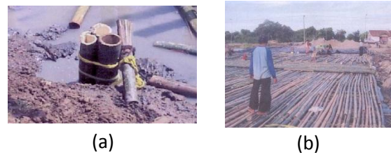
Gambar 2. (a) Cerucuk bambu. (b) Matras bambu (sumber: Irsyam, 2007)
